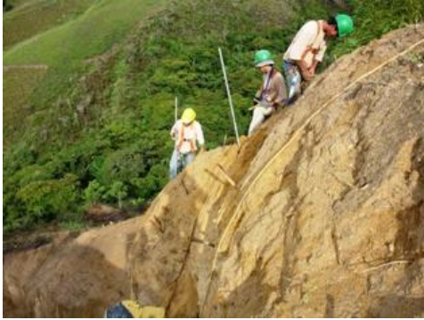
Photo 11 Start the reprofiling
