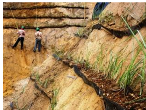
Photo 14: Retained by the mesh substrate
