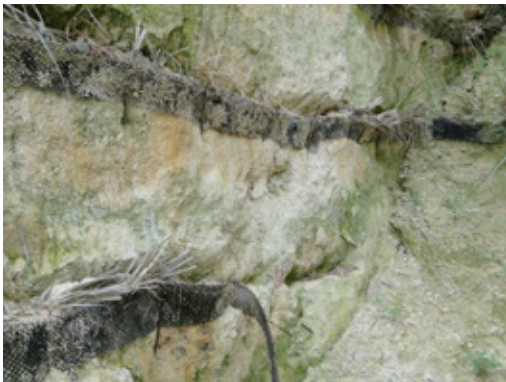
Foto 15: Failure observed in fatigues
