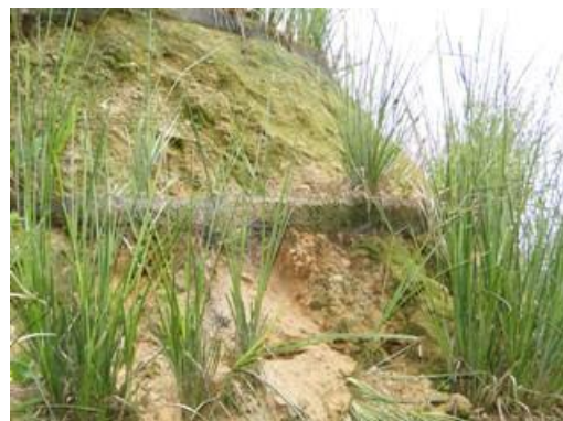
Foto 16: Material retained by the barrier shot lower
