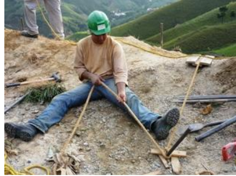
Photo 12 Securing the fall of a worker
