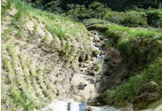
Photo 26: The gully bed collapsed
