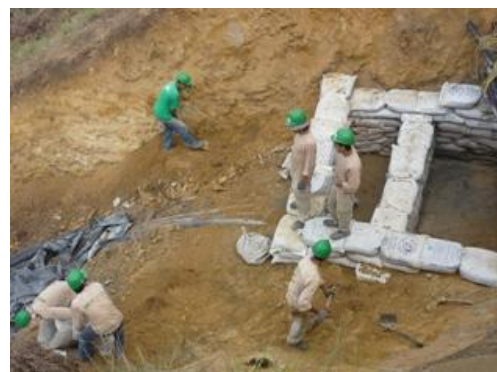
Photo 10 Transition Tanquilla and hoses
