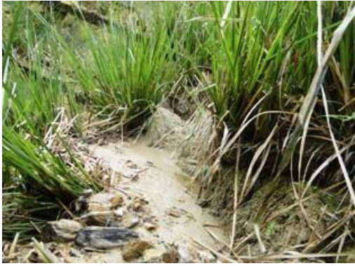
Photos 21 and 22 sediment trapped by the barriers placed in the bed of the gully (May 2010)
