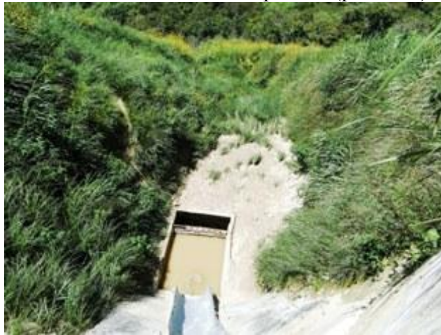
Photo 23. State of the gully in October 2010.
